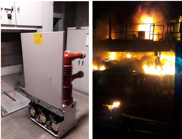
Figure 7: VD4-AF Pilot installation
