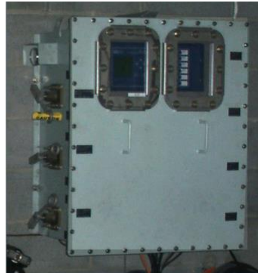
Figure 9. Typical Submersible Control
