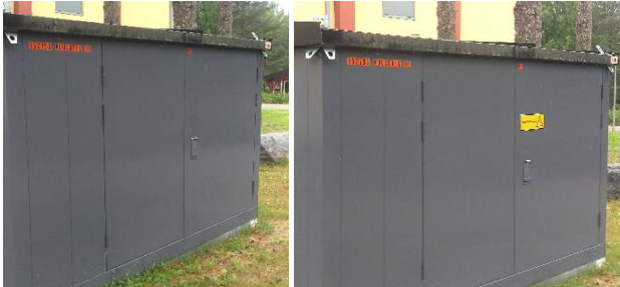
Image 1. Correction of safety markings
