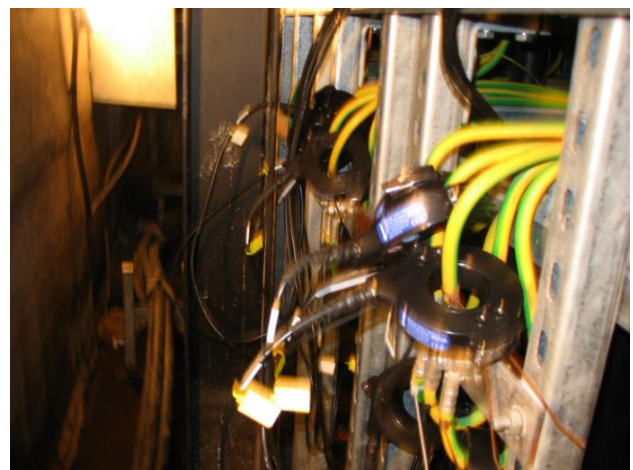
Figure 4 RFCTs Installed Around Cable Earth Straps at Skegoneill Substation
