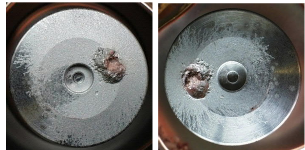
Figure 2: Modification of the surface of vacuum interrupter contacts due to making operations.
