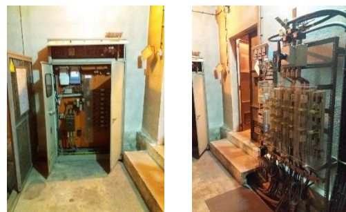
Figure 2 – Power transformer with two smart meters
