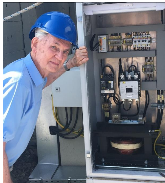
Figure 4. The installed additional coil
