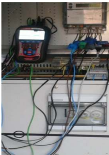
Fig. 2. On site voltage quality measurement.
