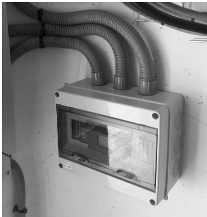
fig. 1 PQ device inside plastic housing.
