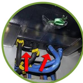
**Figure 6.** Real case of tampered-meter detection
