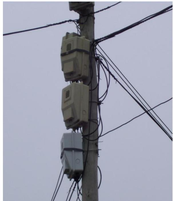
**Fig 1** Height installation of self – administered meters in cabinets
