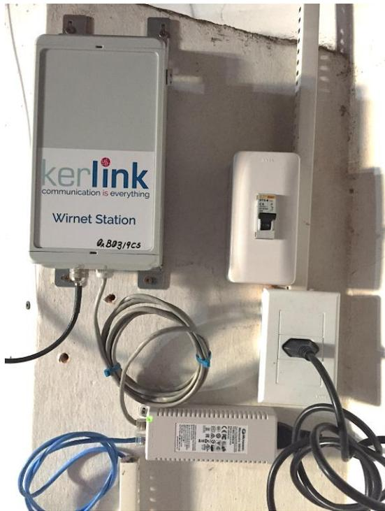
Fig. 4. Kerlink Wirnet Station LoRaWAN gateway installed at Sulgipe building
