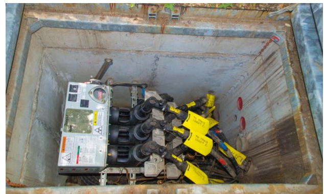
Figure 1: Underground application – showing a Solid dielectric switch installed in a vault.
