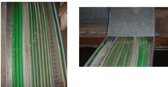
Figure 3 - Example of parallel conductors feeding a cooling
