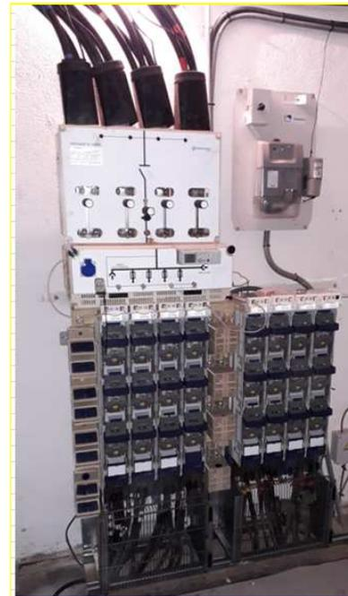
Figure 3. Eight feeders smart LV switchgear
