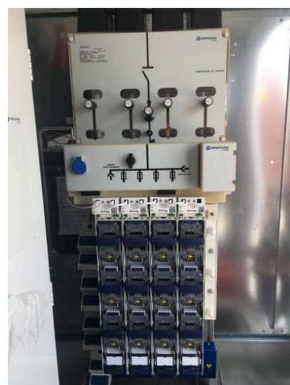
Figure 4. Four feeders Smart LV switchgear
