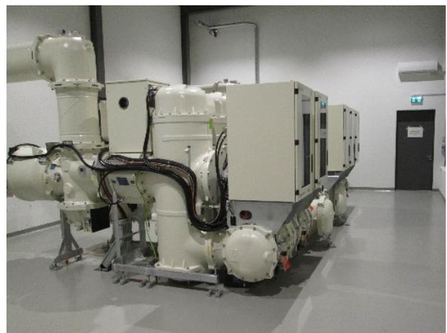
Fig. 1: 145kV g<sup>3</sup> GIS Substation after handover by AXPO, Switzerland early December 2017.
