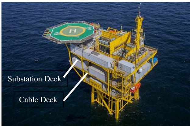
Figure 8: Converter platform in Trianel Wind Farm, Borkum. Photo: Trianel
