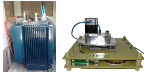
Figure 3. Smart Transformer and its OLTC.
