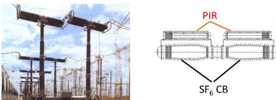
Figure 2. SF<sub>6</sub> circuit breaker with pre-insertion resistors.
