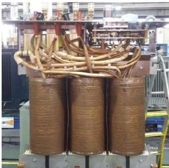
Figure 5. Prototype of a Smart Transformer with integrated PIR in delta (primary side).
