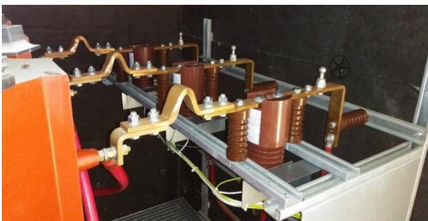
**Fig. 1** MV sensors, provided by ALTEA, installed at the MV busbars of a power transformer
