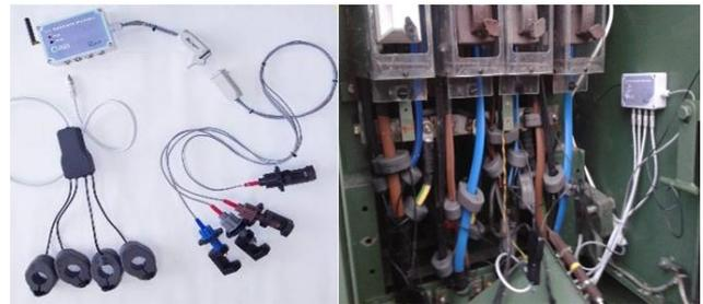
**Fig. 2** LV sensors, provided by MAC, installed at a 4-feeder LV network
