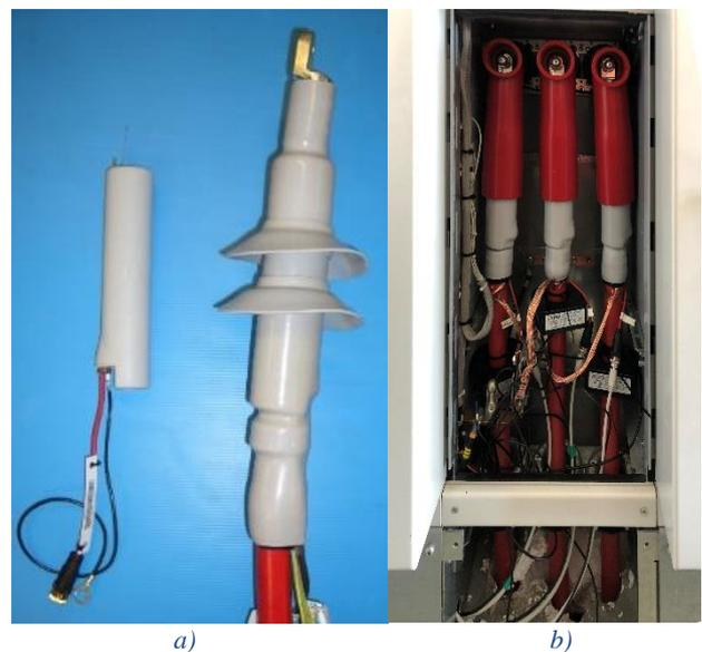
Figure 2a: The QX sensed termination; Voltage sensor (left) and installed termination (right).
