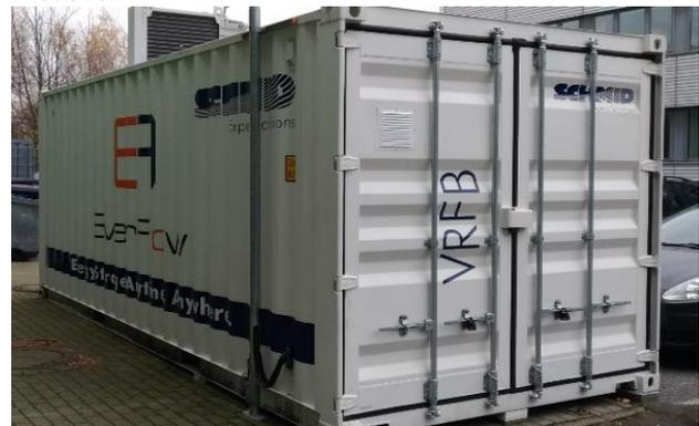
Figure 2 - Picture of the used 30kW/100kWh Vanadium-Redox-Flow-Battery
