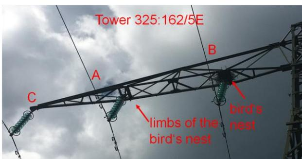
Figure 7: Picture of the tower with bird's nest. The distance to the tower corresponds to fault location result
