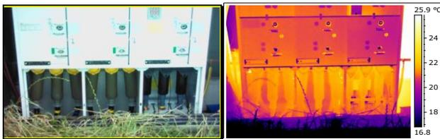
Figure 3. Example of IR image acquired during inspection of RMU on 29.09.2016.
