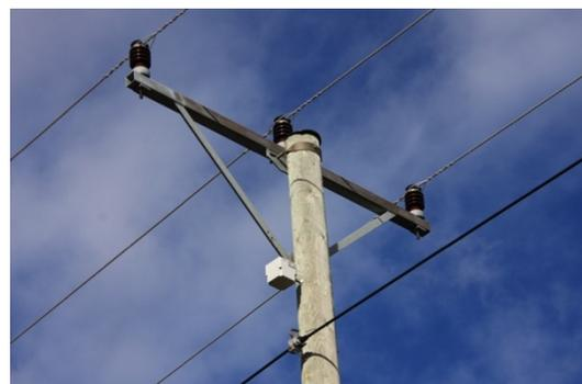
Figure 2: QiC mounted on pole
