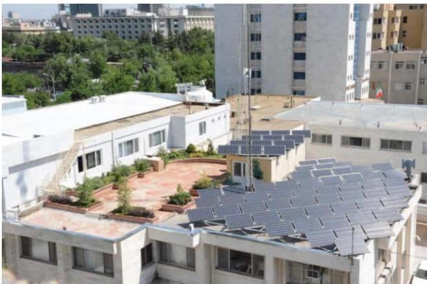
Fig. 2. Mehrsun micro-grid solar panels arrangement.
